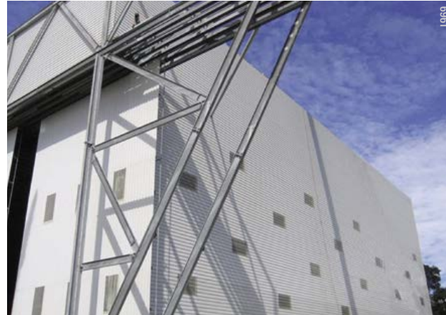
Outriggers allow for clear span door openings.
