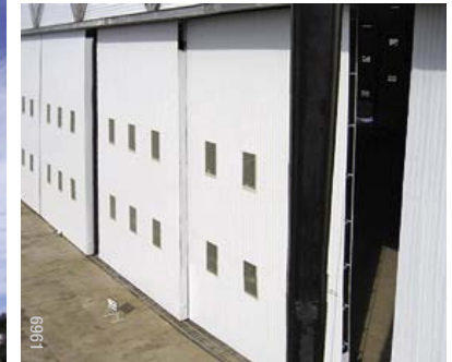
Outriggers allow for clear span door openings.
