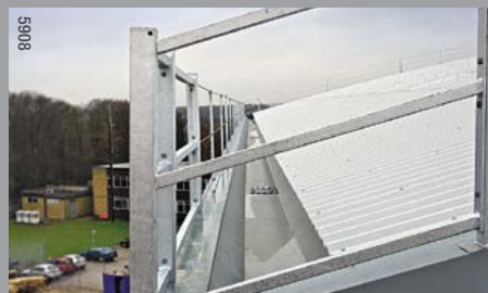
Permanent roof edge protection system with walkable gutters for workers both during construction and for future inspection and maintenance.
